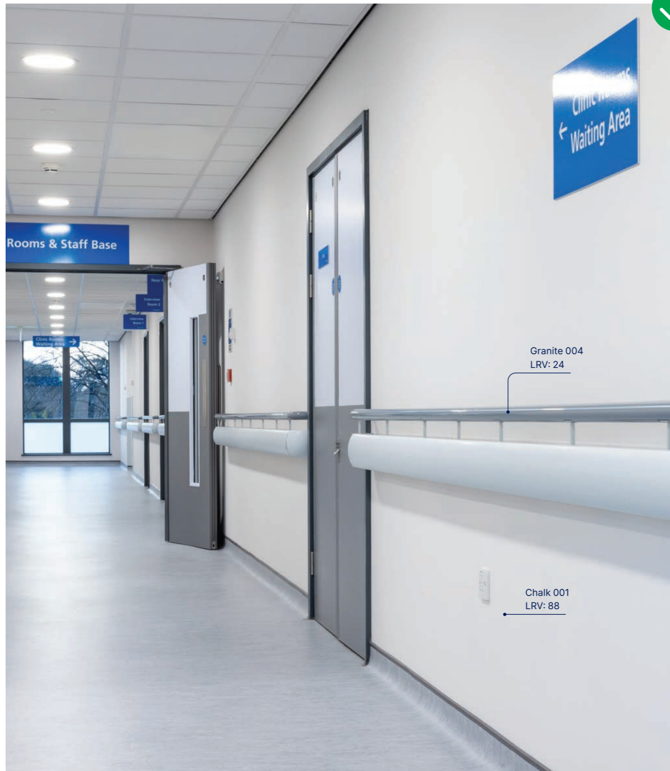
Image shows 30 LRV points difference between the handrail and wall
