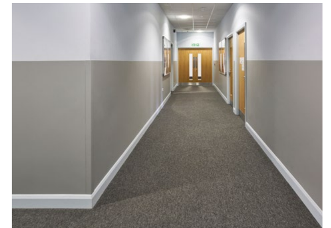
Client: Nottingham Free School Solution: SureProtect Endure Wall Cladding, Surface Mount Standard PVC-u Tape on Corner Guards
